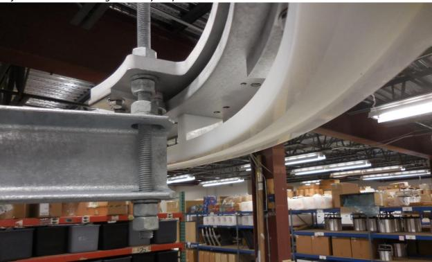
A precision level should be placed across the top of the fixed ring to be sure the ring assembly is level in all directions. You can either adjust the 3 arm mount or the nuts on the threaded rod to make the ring assembly level. Verify it is level in all directions.
